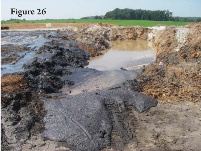
An unlined pit containing petroleum products next to pits which were closed without removing liners and filled with drilling waste and debris.
