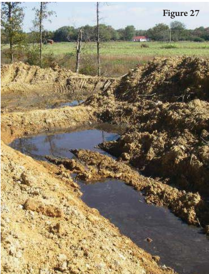
One week after ADEQ discovered fluids overflowing from a pit, the discharged fluids had not been recovered and no one was on the site.
