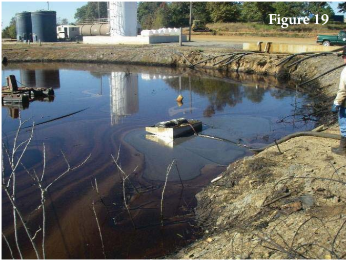
A holding pond for waste that can be disposed of by land application was contaminated by a tank of oil and toxic drilling waste, which must be put into injection wells.
