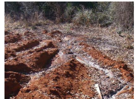
Sediment erosion from a drilling pad.
