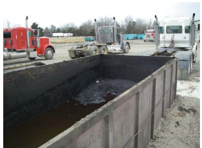
Unpermitted drilling mud bin.
