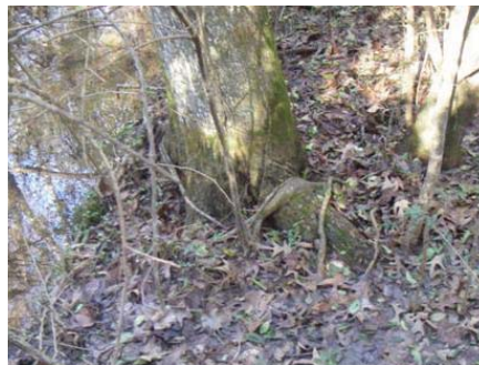
Sediment from a pad runs to a creek, shown in the upper left of photo.
