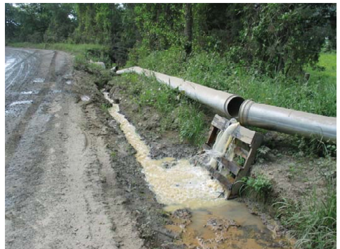
A pipe running from a well pad discharges fluid into a drainage ditch.
