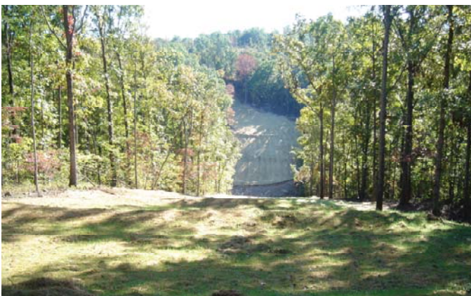
A remediated slope with Best Management Practices in place: stabilized, seeded and with water bars to minimize erosion.
